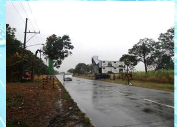
Figure 7: Greenfield Parkway (towards Sta. Rosa – Tagaytay Road)
