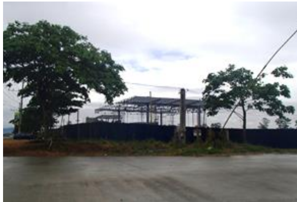
Figure 19: Petron Gas Station (under construction)
